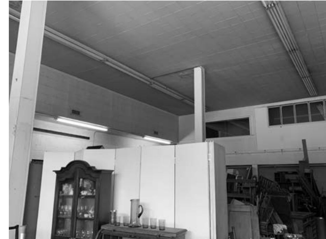
INTERIOR - STORE SIDE FACING NORTH
