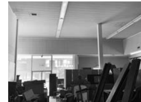
INTERIOR - STORE SIDE FACING SOUTH
